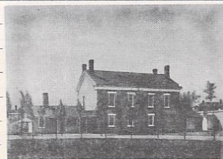
The Old Endowment House
